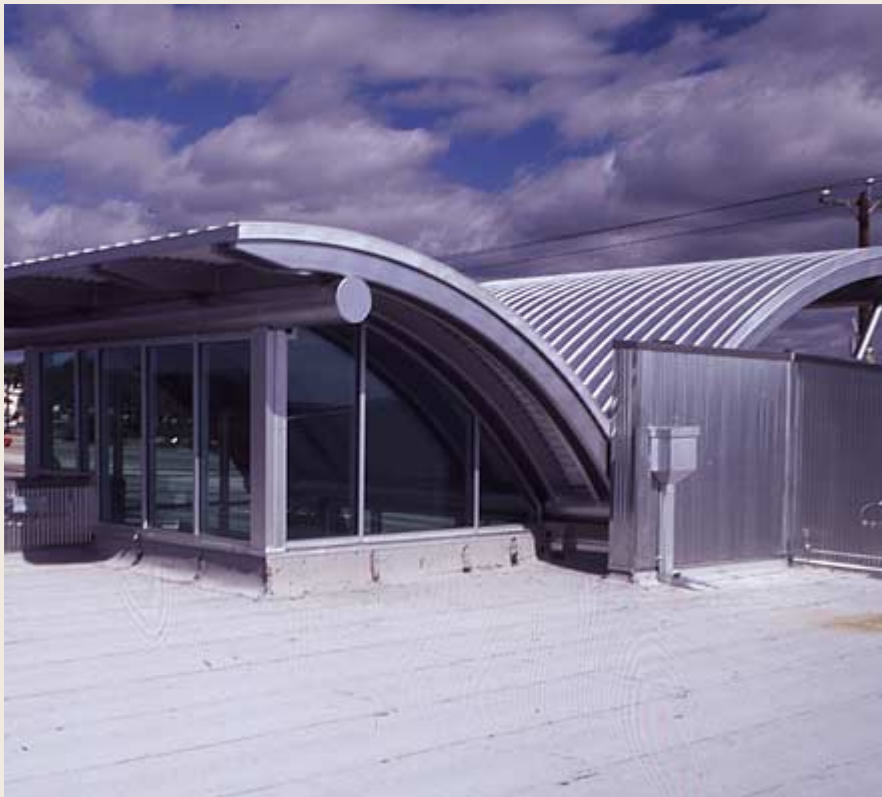
This metal roof, designed in the shape of a seagull, was custom fabricated on site to match the radius of the roof deck atop the headquarters of an electronics retailer. At the curve, where the "wings" meet, Beldon Roofing flashed an internal gutter to drain through the concrete wall. They also installed an SBS modified bitumen system over insulation on the main, low-slope roof section.
