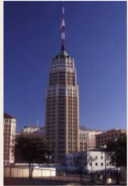
Beldon Roofing used a cold-process modified bitumen system on the Tower Life Building, a San Antonio landmark located in the heart of downtown. Each of the building's many columns required expert workmanship to maintain watertightness.
